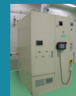
On-site fluorine generator
